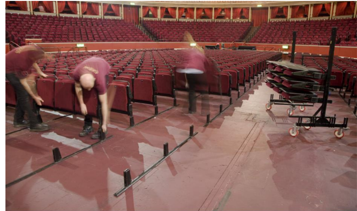
Figure 4 Proposed removable seating (shown being deployed in The Royal Albert Hall, London)
